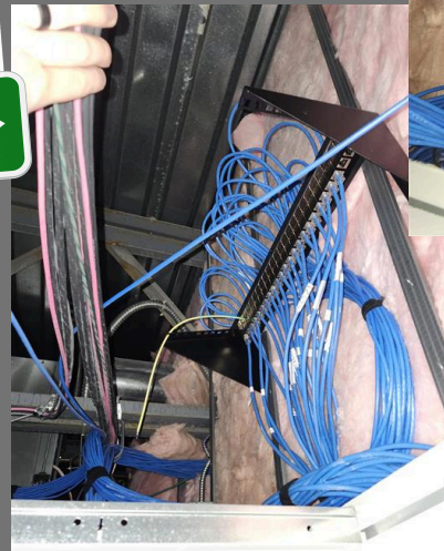
Pictured above: newly installed patch panels
