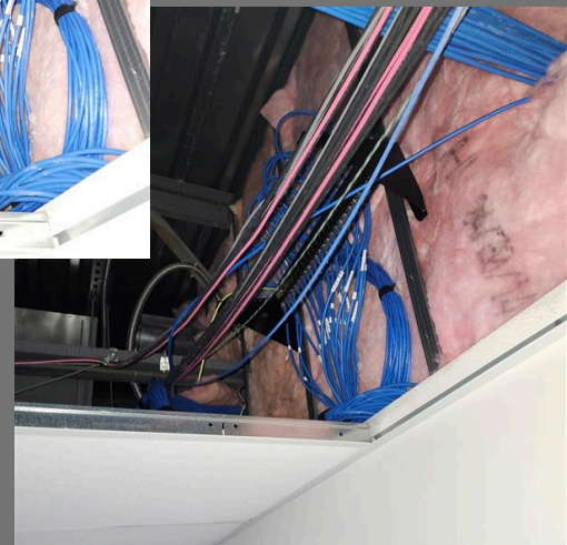
Pictured above: newly installed patch panels
